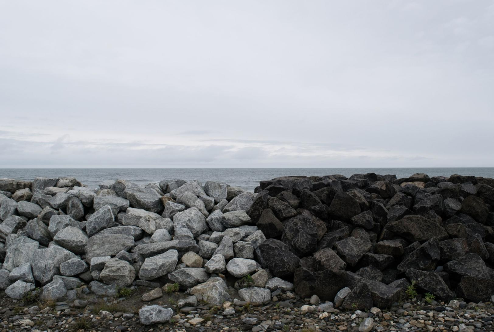
The US Army Corps of Engineers constructed a rip rap sea wall to protect much of Shishmaref from 2005 to 2009. The project is the latest in a number of sea walls constructed to try to slow the rate of erosion on Sarichef Island. *Photo credit: Eli Keene.*
